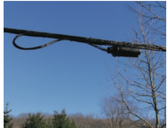
Aerial Fiber Deployment
