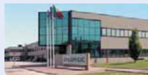
Bologna, Italy UPS manufacturing, R&D centre International sales HQ
