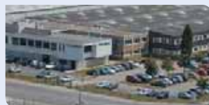
Lyon, France Industrial UPS manufacturing R&D centre
