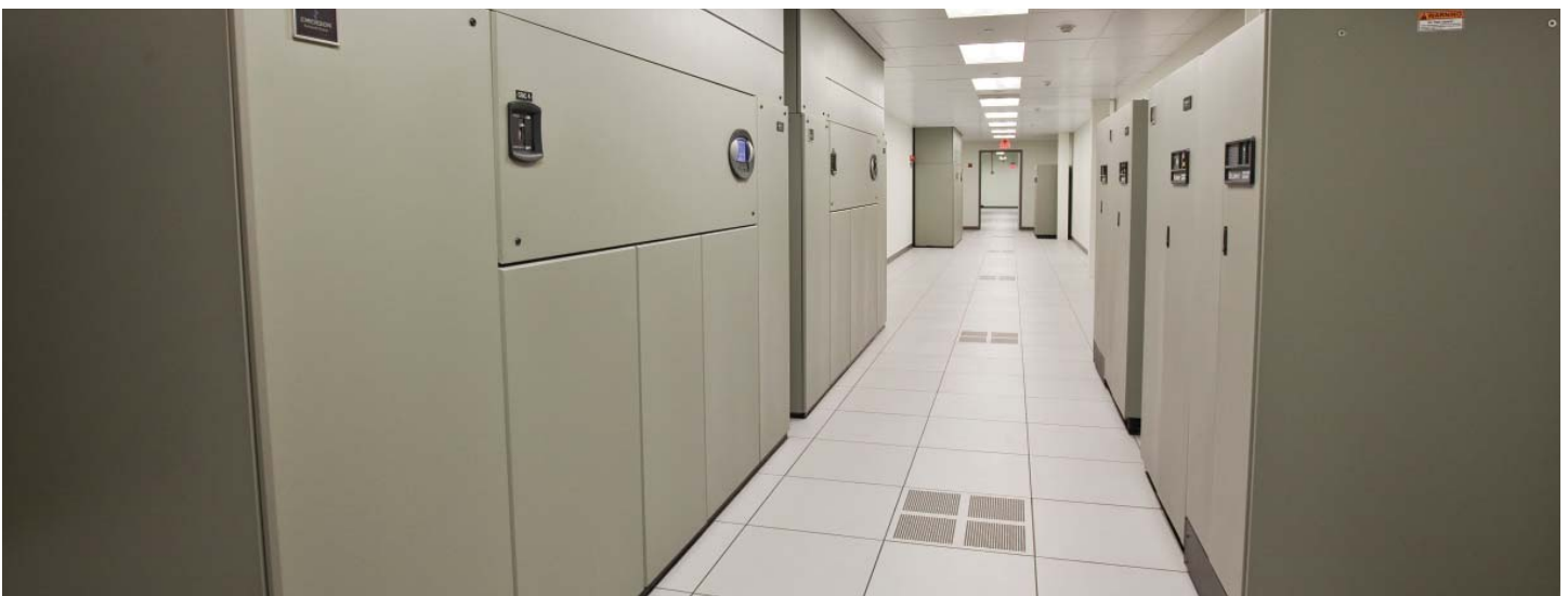
Liebert DS™ precision cooling systems from Emerson Network Power provide efficient, precise, reliable control of room temperature, humidity and airflow for proper operation of critical electronic equipment.
