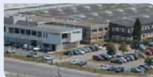
Lyon, France Industrial UPS manufacturing R&D centre
