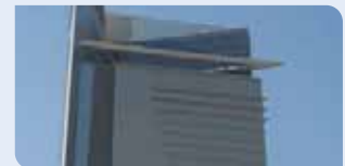
Dubai, UAE Middle East HQ
